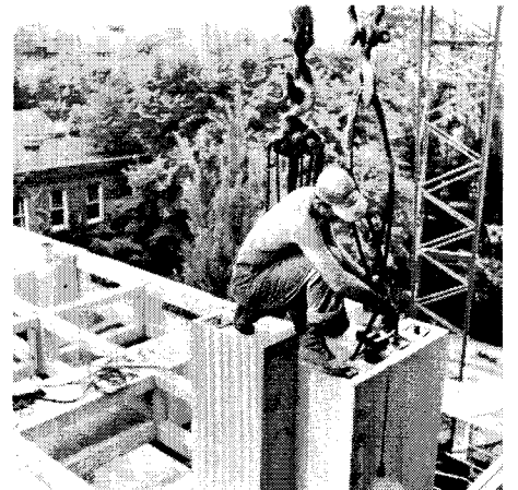
Fig. 6. Construction photos by Marshall D. Meyers of Kahn's office showing connection of main beams with columns and (right) post-tensioning cables in columns. Often overlooked, the use of pre- and post-tensioned concrete members represented one of the first major uses of these techniques in architectural settings. (Copyright 2003, Marshall D. Meyers Collection, University of Pennsylvania Historical and Museum Commission.)
